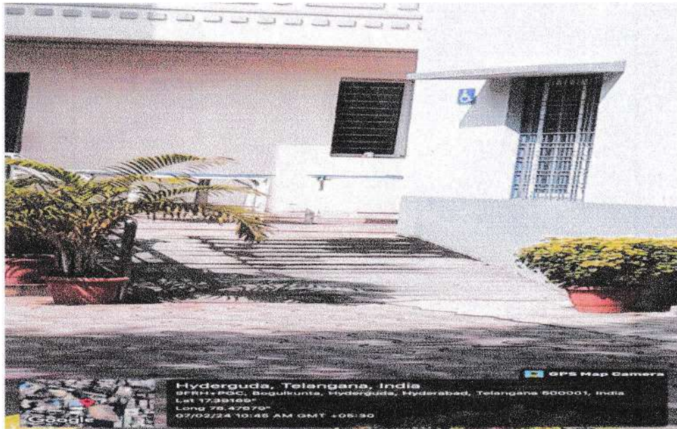
Ramp at 'D' block
